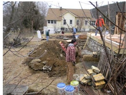
Construction crew hard at work!
