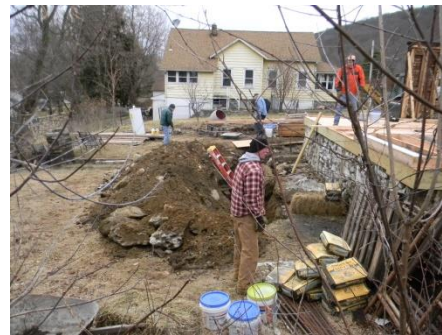
Construction crew hard at work!
